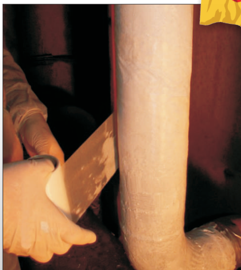
Fiberglass reinforcement tape over 1st coat of ENESEAL CR
