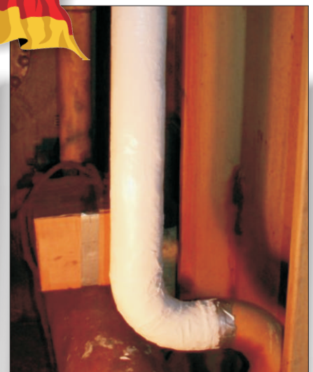
Final coat of ENESEAL CR
