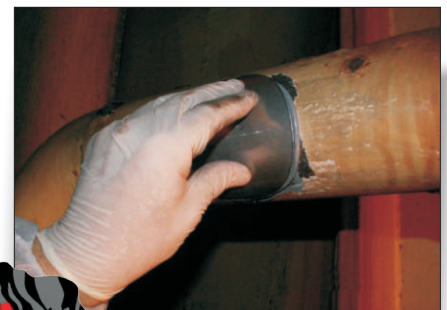
Patch applied to hole
